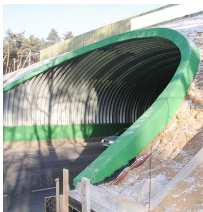
concrete headwall – beveled end.
