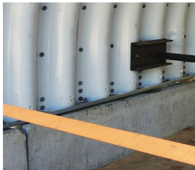
Fig. 8. Connection of the steel structure with concrete foundations
